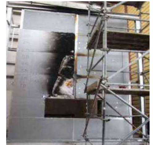
WALL CAVITY IN WALL ASSEMBLY AFTER FIRE TEST
