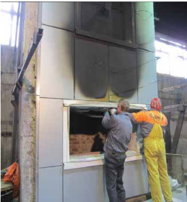
ALUBOND PANELS – REMOVED FROM WALL ASSEMBLY
