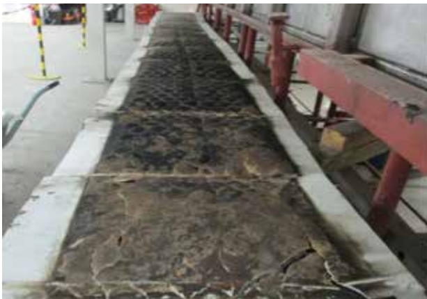
CORE AFTER THE TEST (LOCATED NEAR THE FIRE END)
