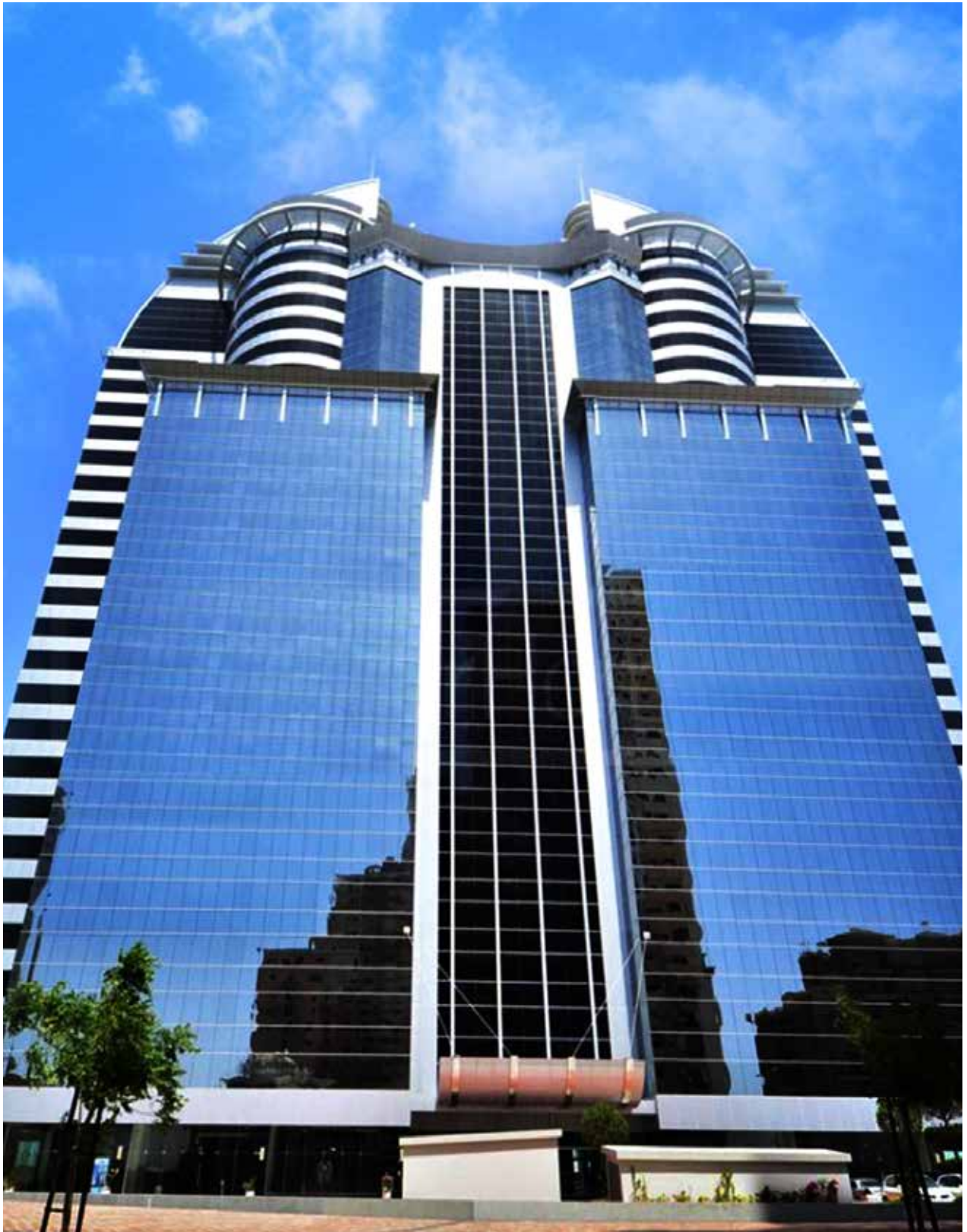
SIT TOWER, DUBAI SILICON OASIS, DUBAI, UAE Contractor: Beijing Emirates Intl. Construction Company. Consultant: Eng. Adnan Saffarini
