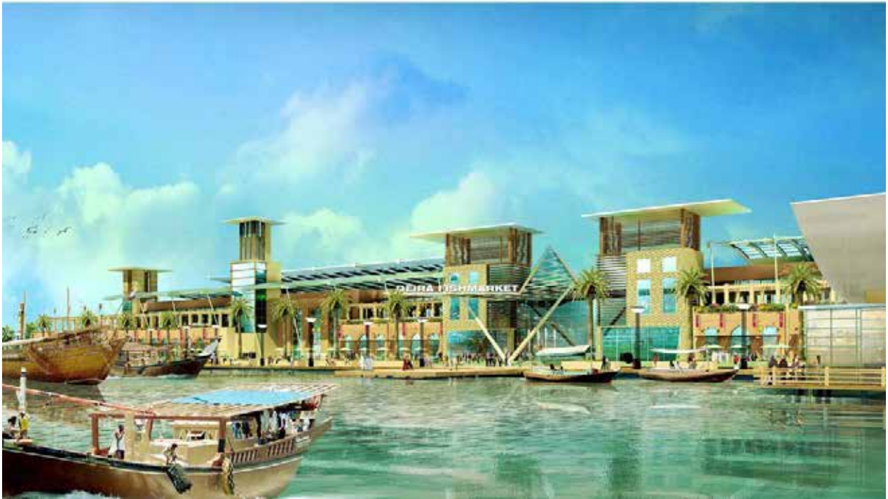
NEW DEIRA FISH MARKET-MIXED USE, DUBAI, UAE Contractor: Bhatia General Contracting Company LLC Consultant: Hyder Consulting Middle East Limited.
