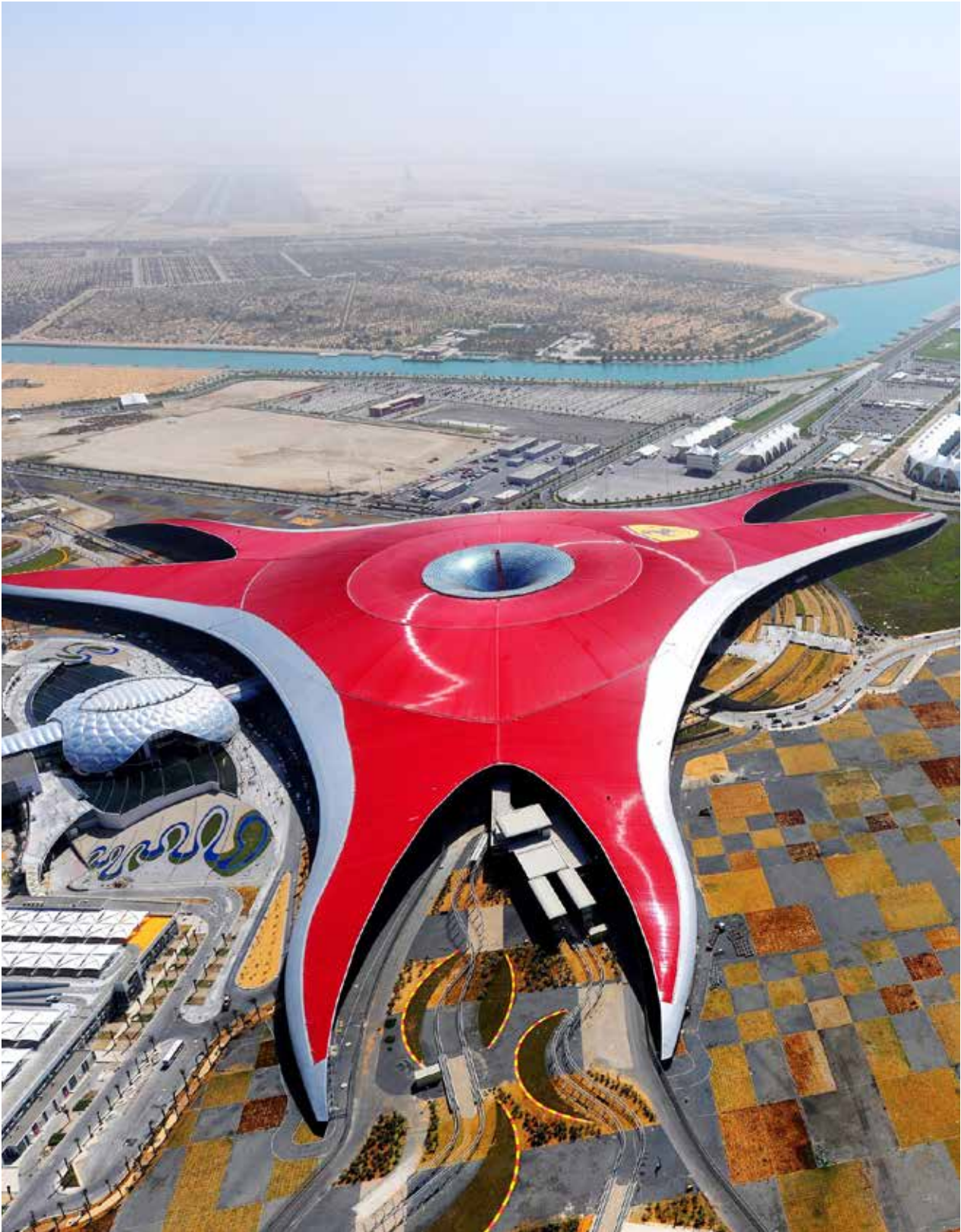
FERRARI WORLD YAS MARINA, ABU DHABI, UAE Contractor: SIXCO
