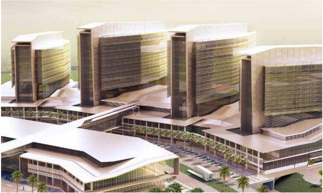
AL MAFRAQ HOSPITAL, ABU DHABI, UAE Contractor: Al Habtoor Leightoor Leighton Group
