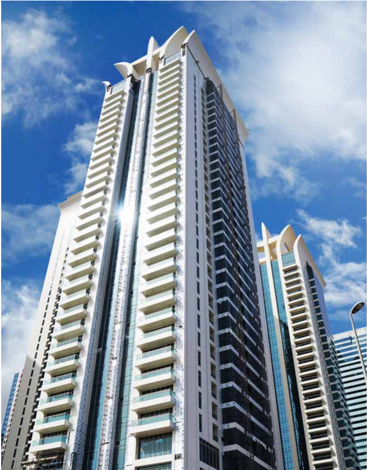
TAMWEEL TOWER, DUBAI, UAE Consultant: ALEC
